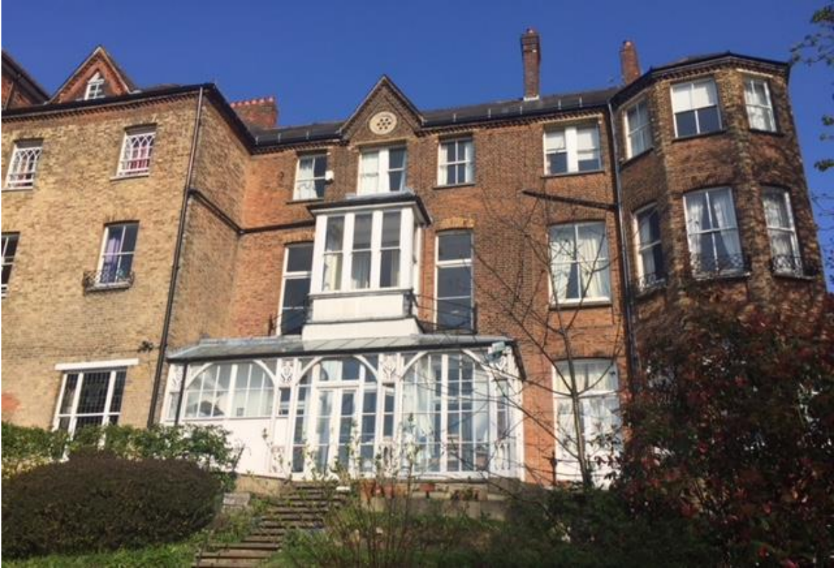
Rear elevation of host building
