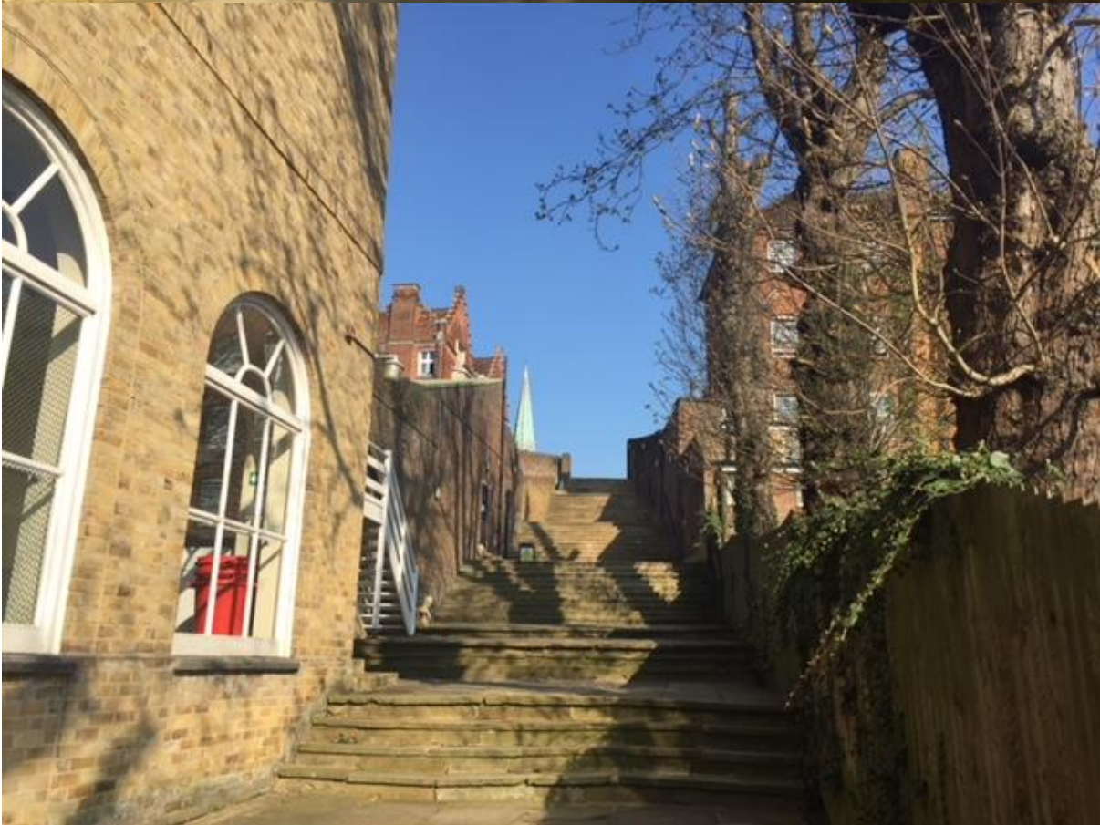
Rear elevation of host building
