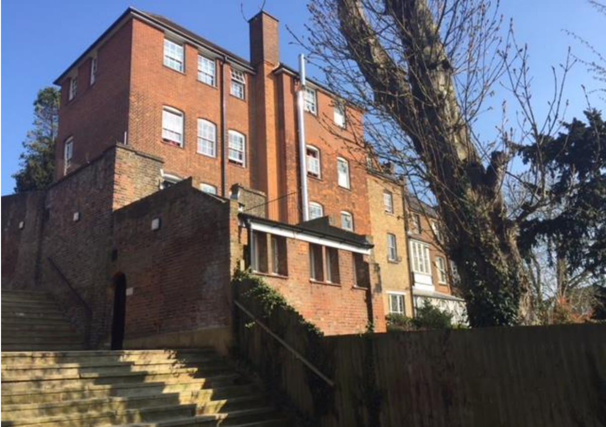
Rear elevation of host building
