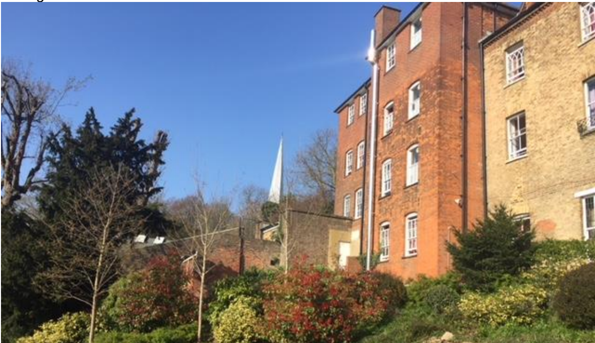
Rear elevation of host building
